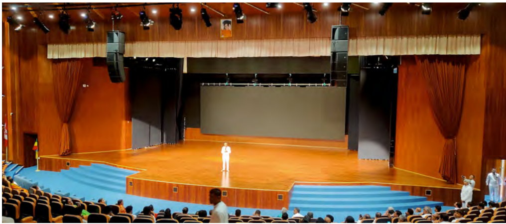
An L-Acoustics A Series system has been installed in the Sai Hira Global Convention Centre
